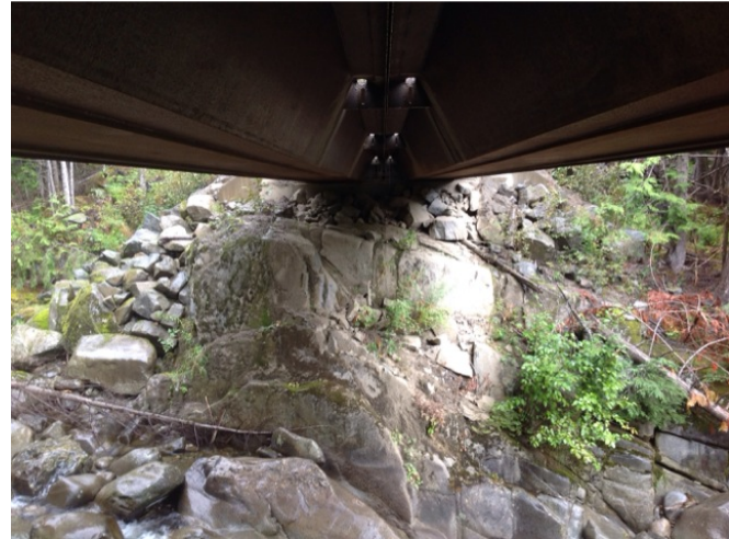
Left Bank Abutment when facing downstream
