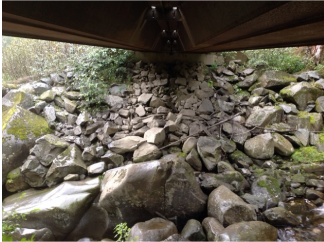
Right Bank Abutment when facing downstream
